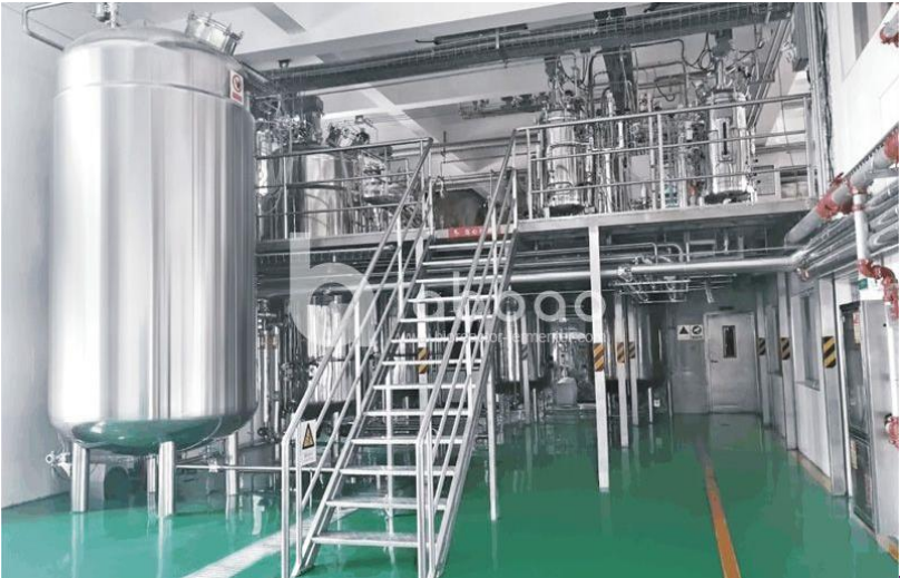
Low environmental impact production center
